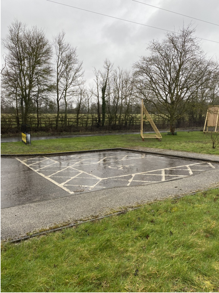
Accessible parking spaces.
