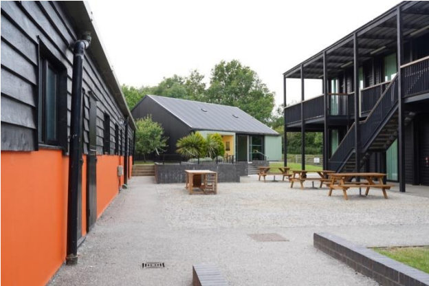
Stableblock, reception and main studio building
